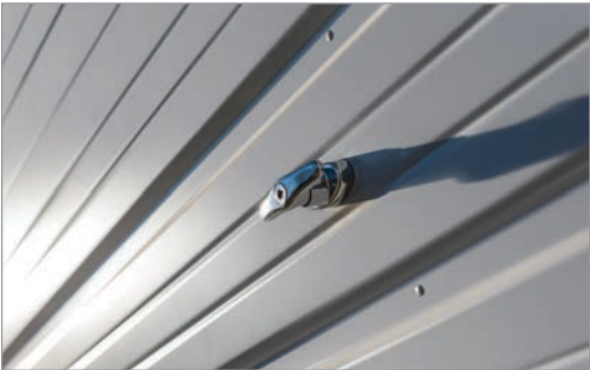
Two horizontal ribs with alternating 'v' grooves
